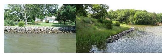
**Breakwater:** Offshore shore-parallel structure that reduces the wave energy reaching the beach and supports sediment accretion landward of the structures. Commonly used in combination with sand nourishment to create or enhance an existing beach. Breakwaters are distinguished from rock sills by the size of the structures, distance offshore, and presence of a sand beach instead of a tidal marsh landward from the structures.
