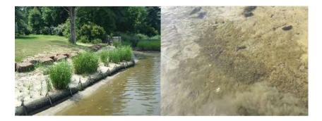
**Loose Shell:** Mounds of uncontained shell placed nearshore to reduce wave energy.
