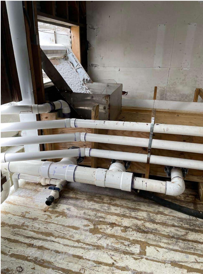
This picture shows PVC piping for circulating brine solution.
