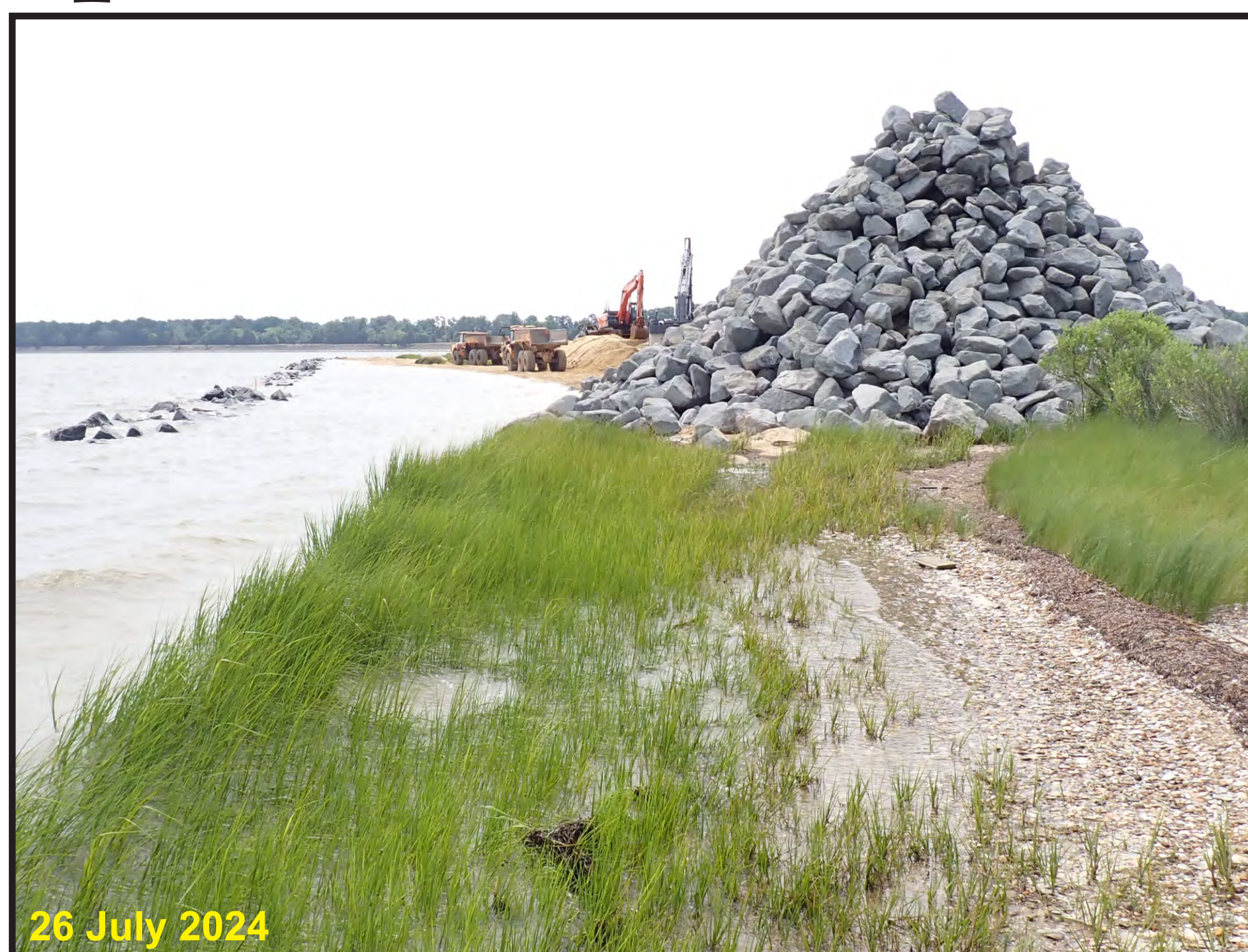
Stockpiled materials were moved by construction equipment along the shoreline. The large pile of armor rock was placed along the shoreline where sill construction is underway in the nearshore.
