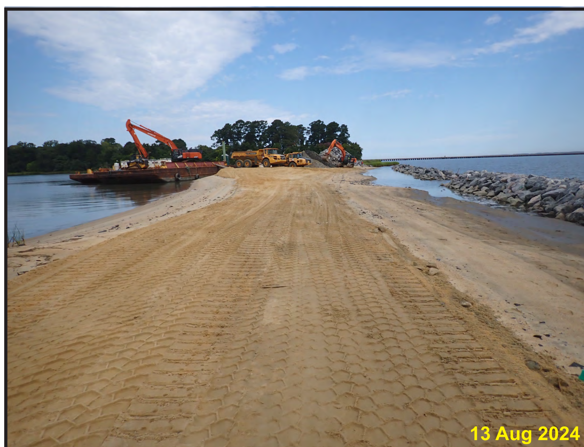
The gap between the existing spit sections was filled with sand and sills and breakwater constructed.
