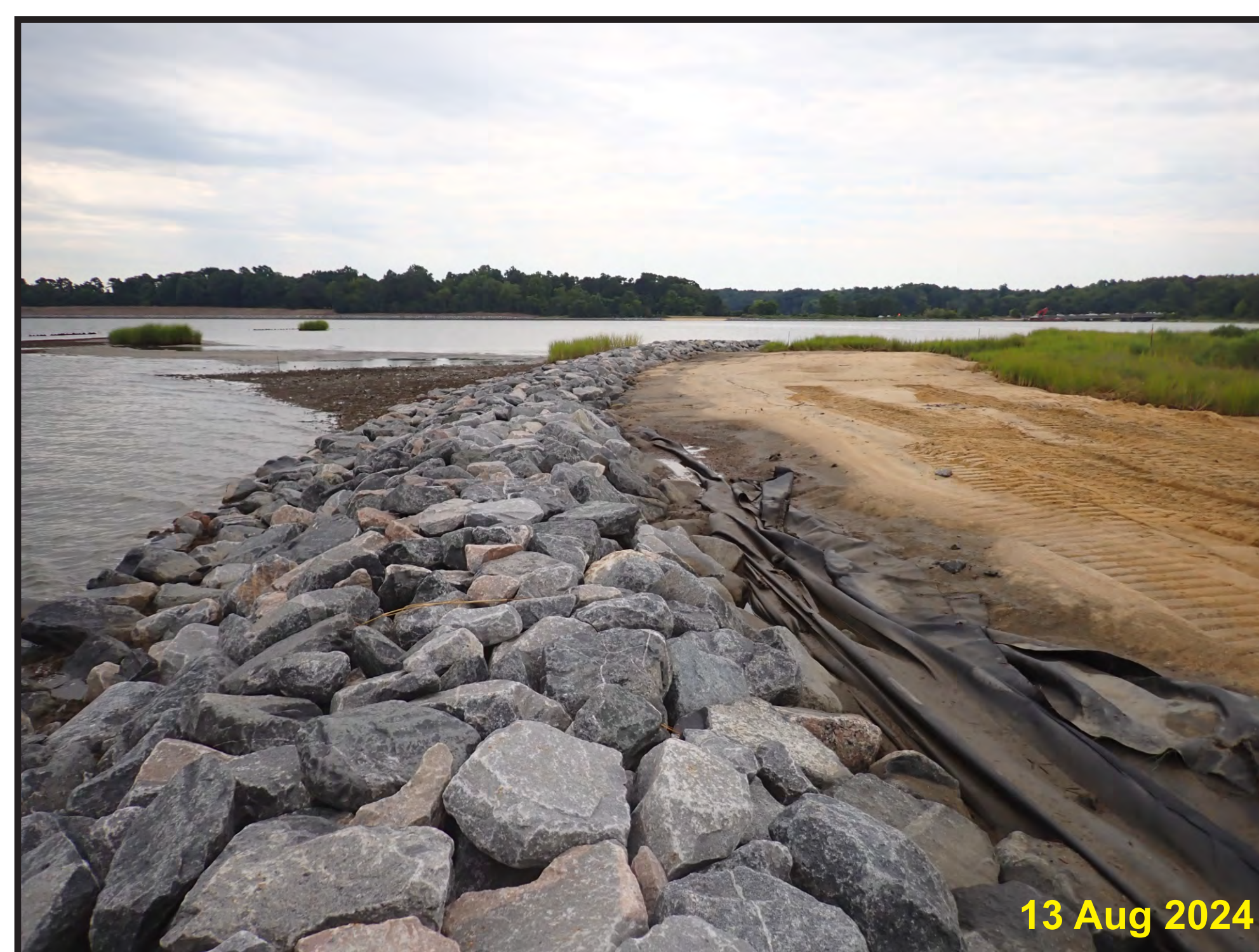
Complete sill on the eastern end before sand was planted.
