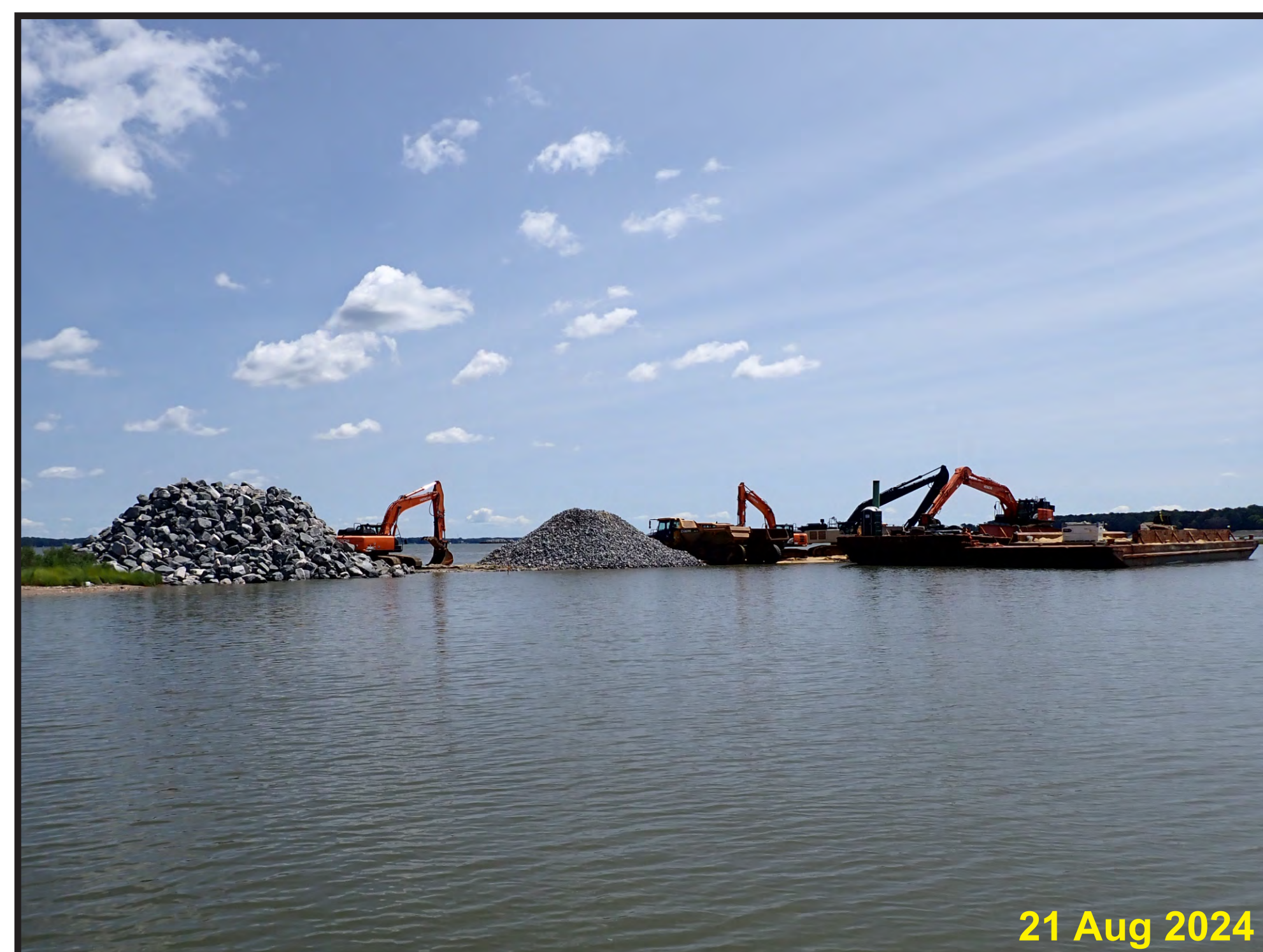
Materials were brought in by barge and stockpiled on site.
