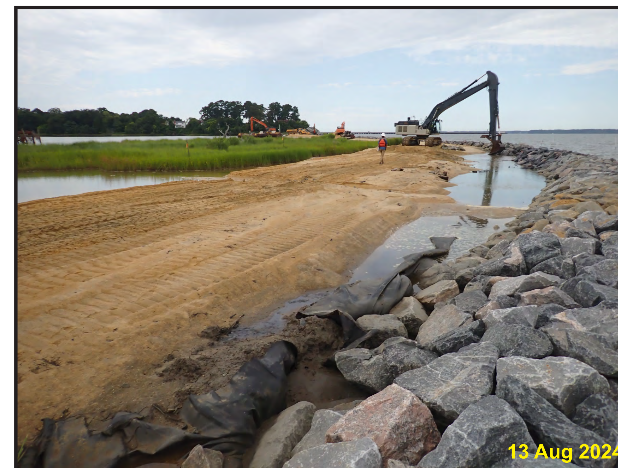
Sill construction is complete along this eastern section of the shoreline. Filter cloth was placed under the structures.
